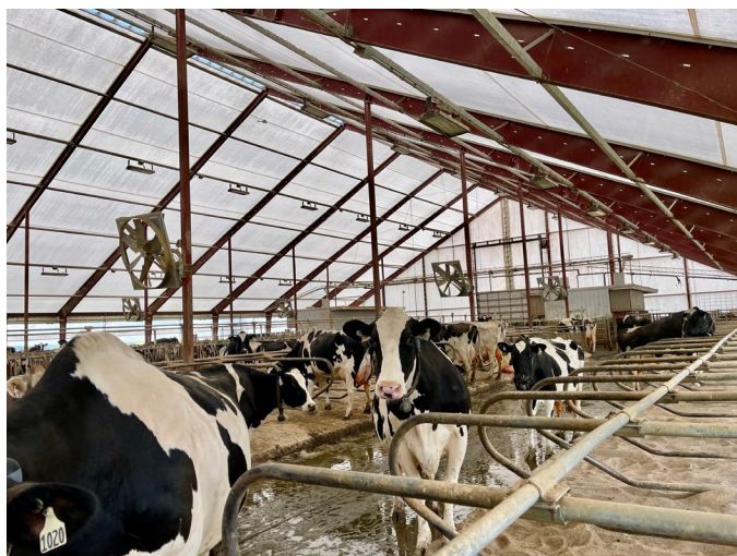
Figure 4. Naturally ventilated fabric dairy buildings. Note the steep 6:12 roof pitch (photo: Nesli Akdeniz)
