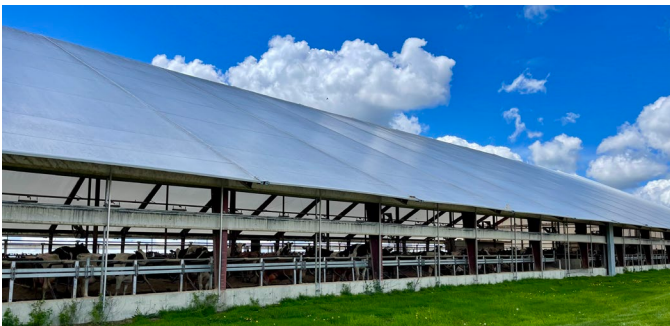
Figure 2. Split sidewall curtains help regulate airflow rates without causing a draft for the cows (photo: Nesli Akdeniz)
