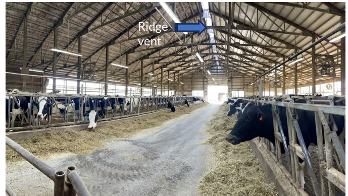
Figure 3. The ridge vent is important for removing heat, moisture, and gases. It is the barn's chimney. (photo: Nesli Akdeniz)
